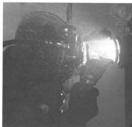
Using pure oxygen gas, this diver can produce a flame hot enough to cut metal underwater.
